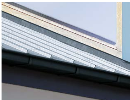
Detail 2: druipranddetail bakgoot
